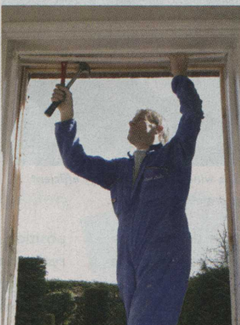
Take out the horizontal parting bead.
