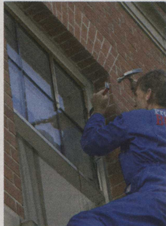
The top sashes were screwed in under the sealed units.
