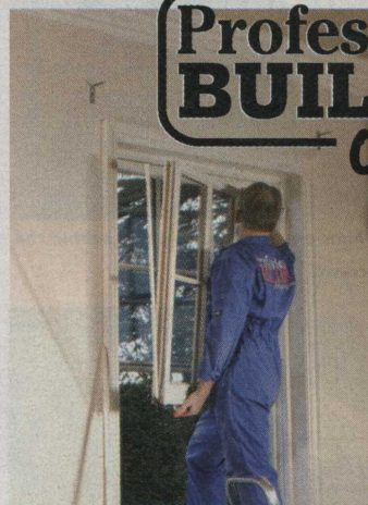
Take out the old sash.
